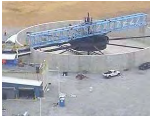
Tank-based pond replacement
