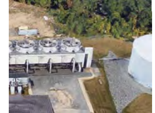
Source water treatment
